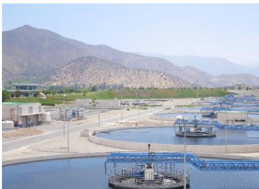
Settlement tanks of La Farfana WWTP
