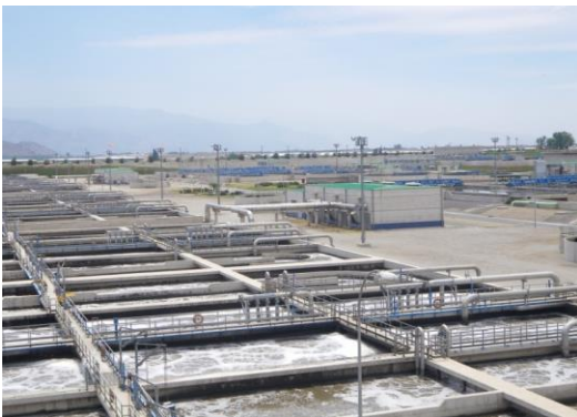
Biological reactor tanks of La Farfana WWTP
