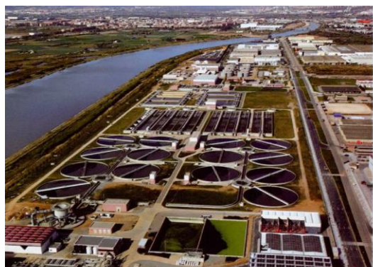
Aerial view of Barcelona Baix Llobregat WWTP
